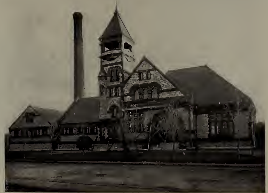
PUMP-HOUSE, BOSTON WATER WORKS, Chestnut Hill.
